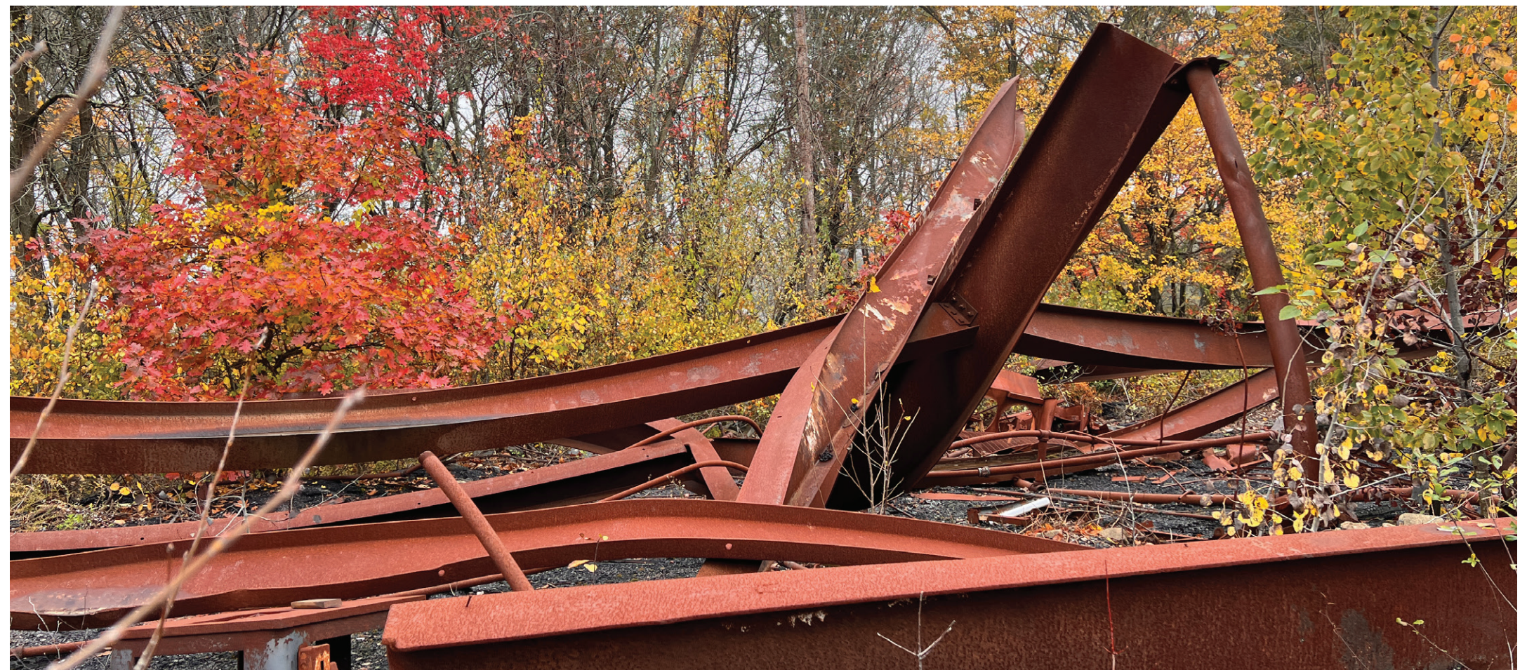
Figure 11: Steel structural members from the pre-existing factory warped and collapsed from the heat of the fire.
